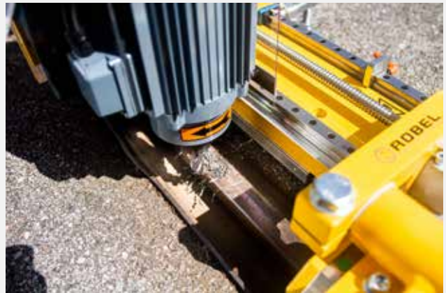
Drainage groove with ROFACE rail milling machine
