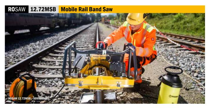
For cutting rails without sparking in new construction and maintenance.
