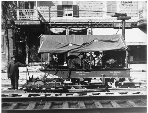
**Fig. 1:** Grinding machine for rail maintenance from the year 1912 in Montreal/Canada
