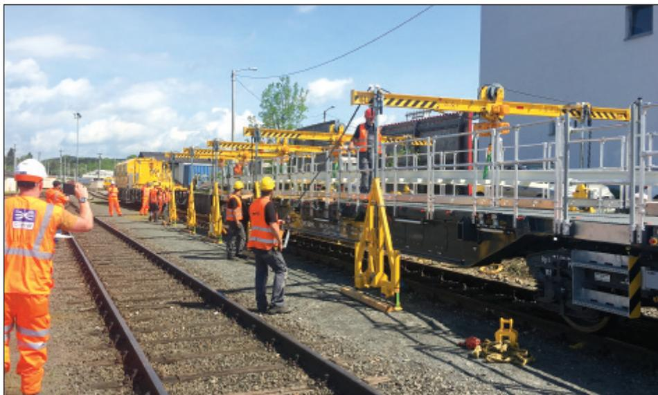
to exchange the switch within the tunnel confines. To make the process more efficient and safer, these electrical gantries came pre-assembled and loaded on a specially designed on-off loading device, a modular unit which secures with twist locks to the platform on Power Car A.
