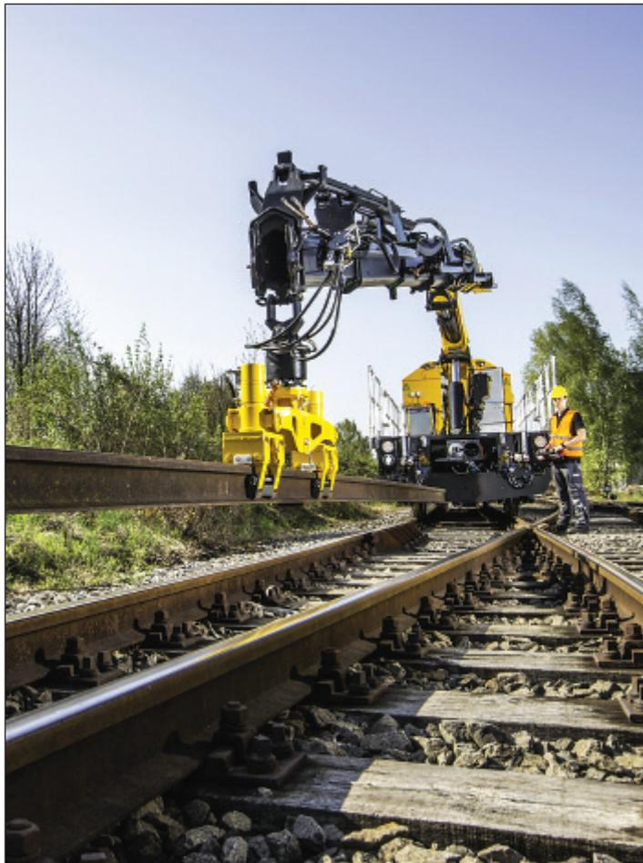
**Above: An 18 metre plain rail exchange in progress as part of Case Study 2 tests.**
