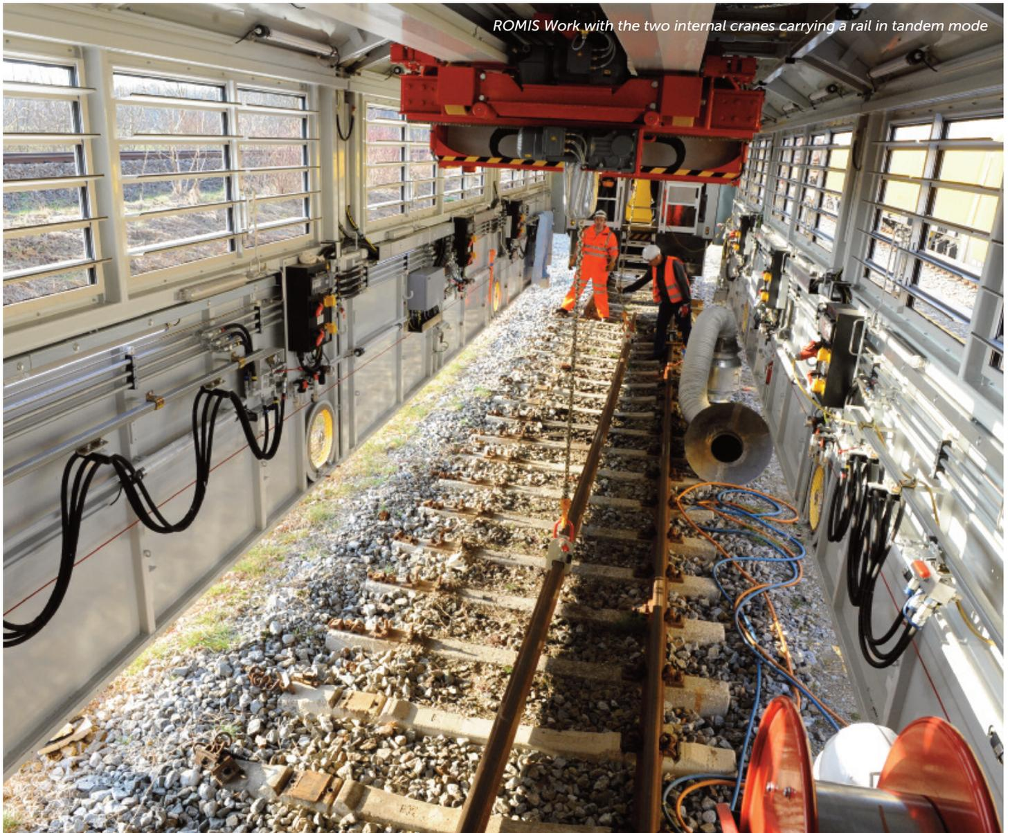
ROMIS Work with the two internal cranes carrying a rail in tandem mode
