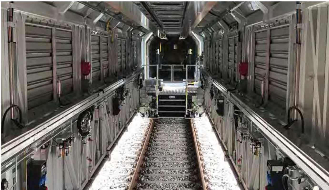
Fig. 4: Work area in the Mobile Maintenance Unit
