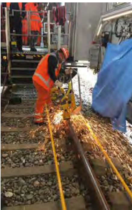
Fig. 7: Rail joint grinding at the trial work site Source DB Netz
